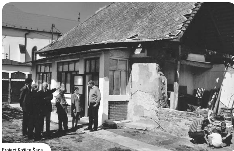
Project Košice Šaca
